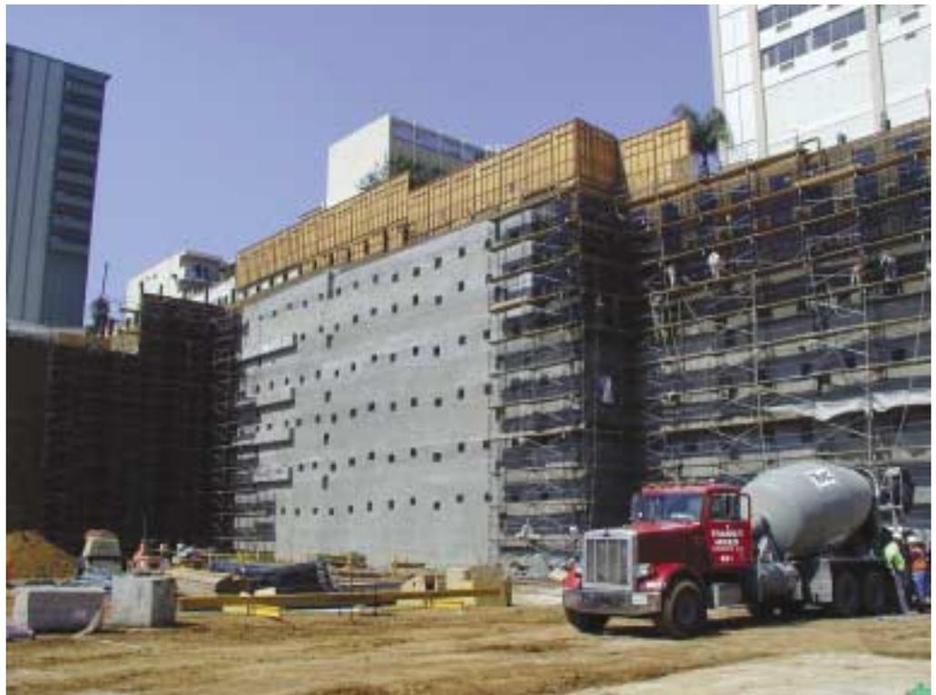
Partially completed Hollywood & Highland project in Hollywood, Calif. This project required over 13,000 yd<sup>3</sup> of 25-in.-thick shotcrete walls. A section of sawcut preconstruction panel for the project showed complete encasement of the reinforcing steel, even with lap-spliced #11 bars
